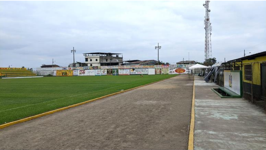
Circuito de footing
